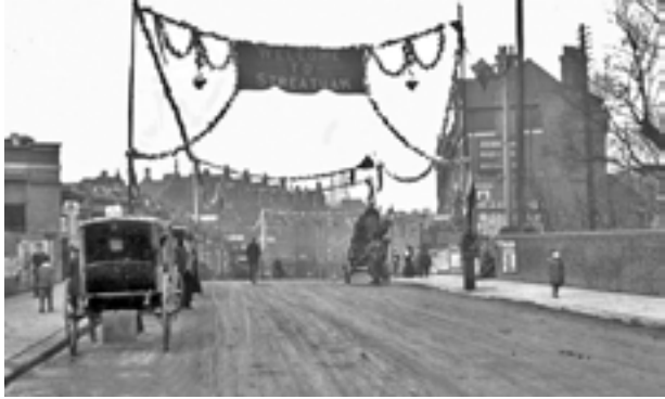
Streatham Station Railway Bridge Christmas 1908
