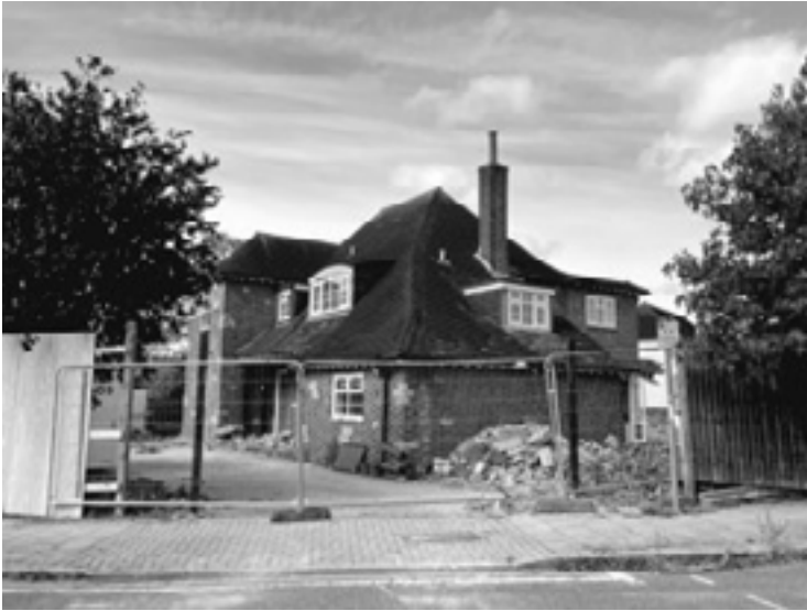
49 Abbotswood Road awaiting demolition
