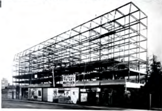
141 STEEL FRAMED FLATS - STREATHAM, LONDON, ENGLAND The first all-welded framework for a block of flats in England.
