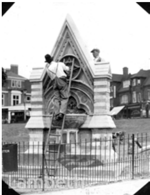
Reassembling the Dyce Water Fountain in its new location on Streatham Green
